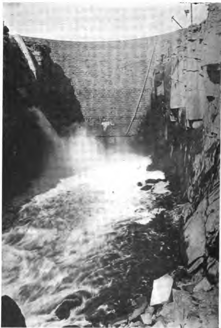
FIG. 228.—Pathfinder Dam, North Platte River, Wyoming. Lower face showing concrete ladder, and 6500 second-feet of water discharging from tunnel.
